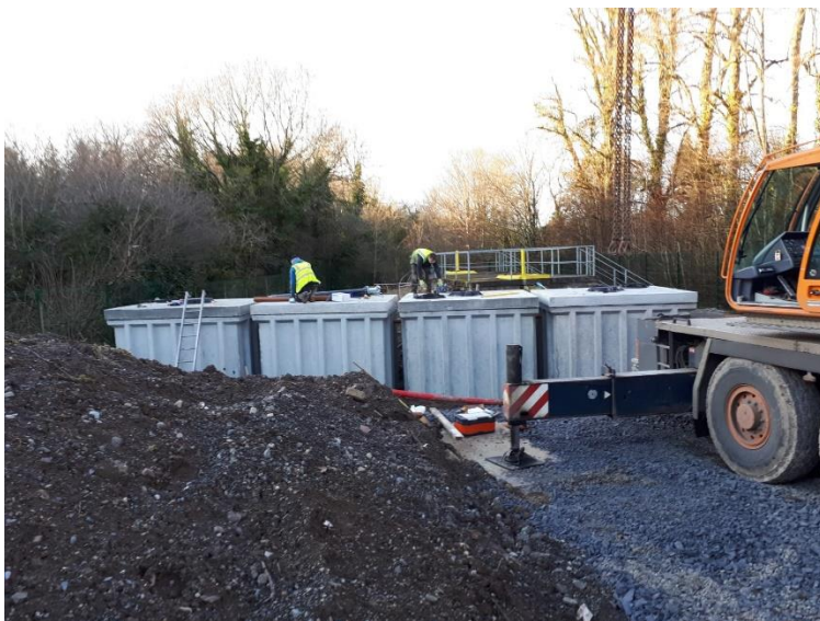
Picture 3. Four new tanks placed at end of 2020
