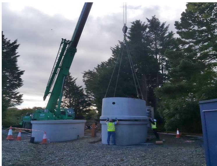
Picture 7. Primary tanks being craned into location.
