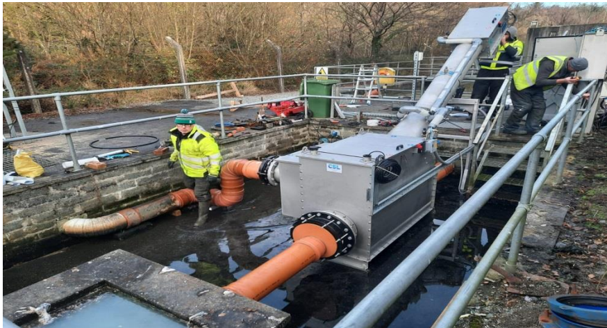
Picture 5. Screen Aughrim WWTP
