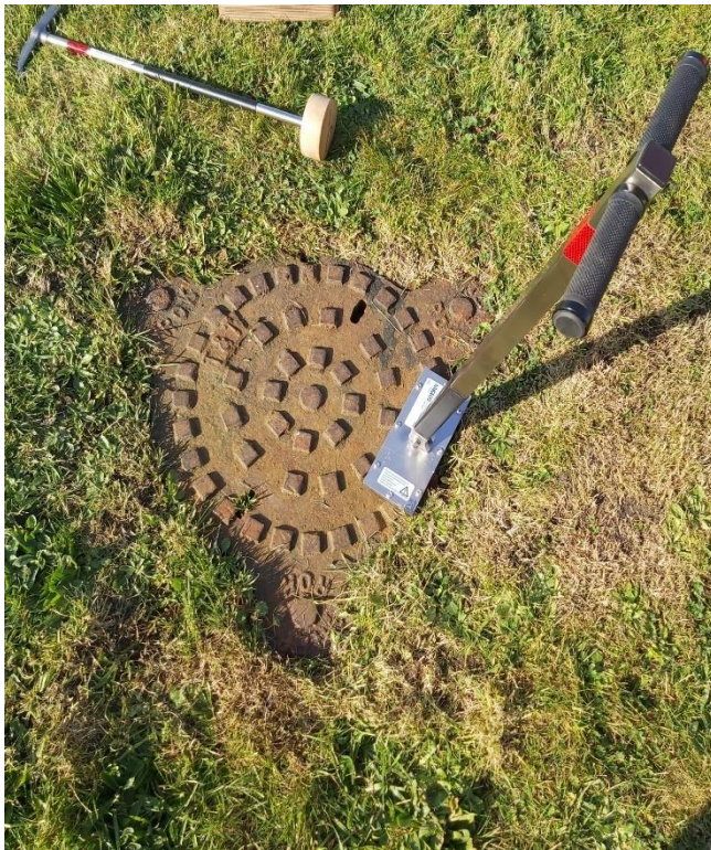
Picture 8. Manhole examination works
