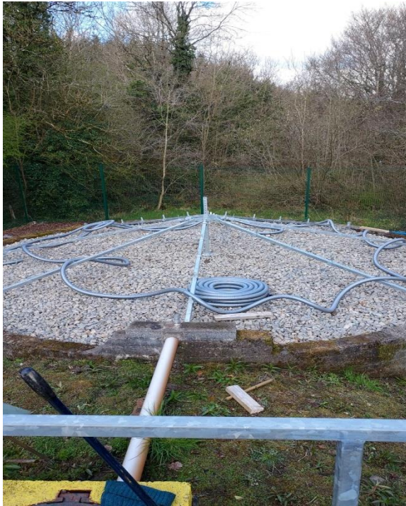
Picture 1. New filter stone placed.
