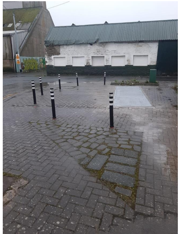
Picture 9. New sump cover at Bond St. Wicklow
