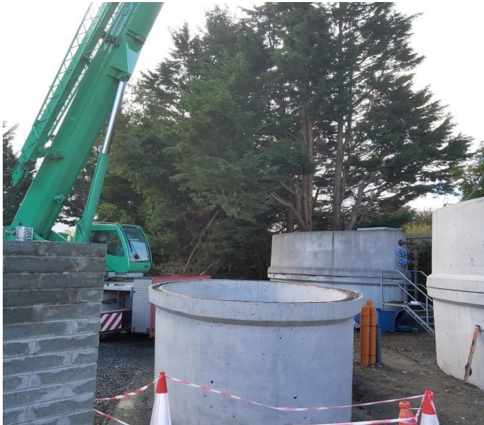
Picture 6. Tanks arriving to site.
