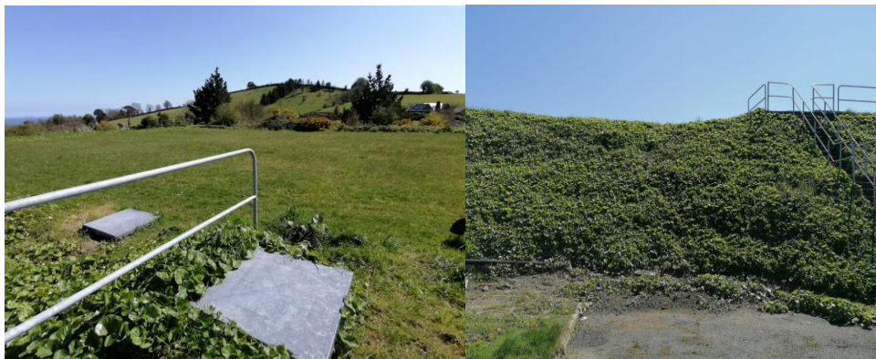
Drummin Reservoir Greystones
